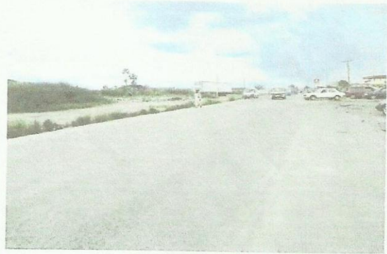
STATE OF THE ROAD AFTER REHABILITATION
