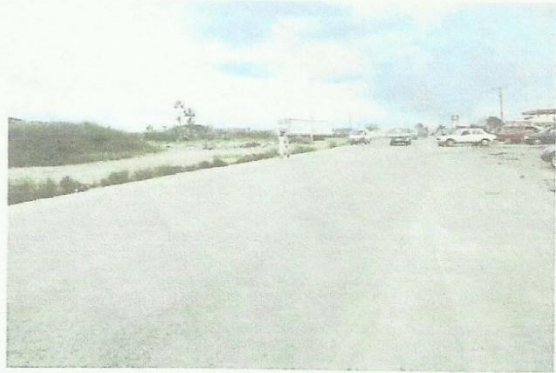
STATE OF THE ROAD AFTER REHABILITATION
