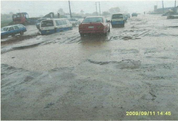
STATE OF THE ROAD BEFORE REHABILITATION
