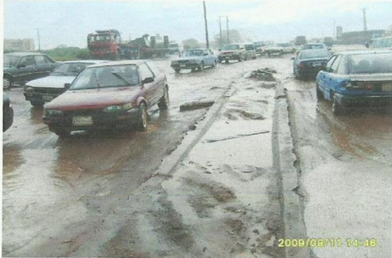
STATE OF THE ROAD BEFORE REHABILITATION
