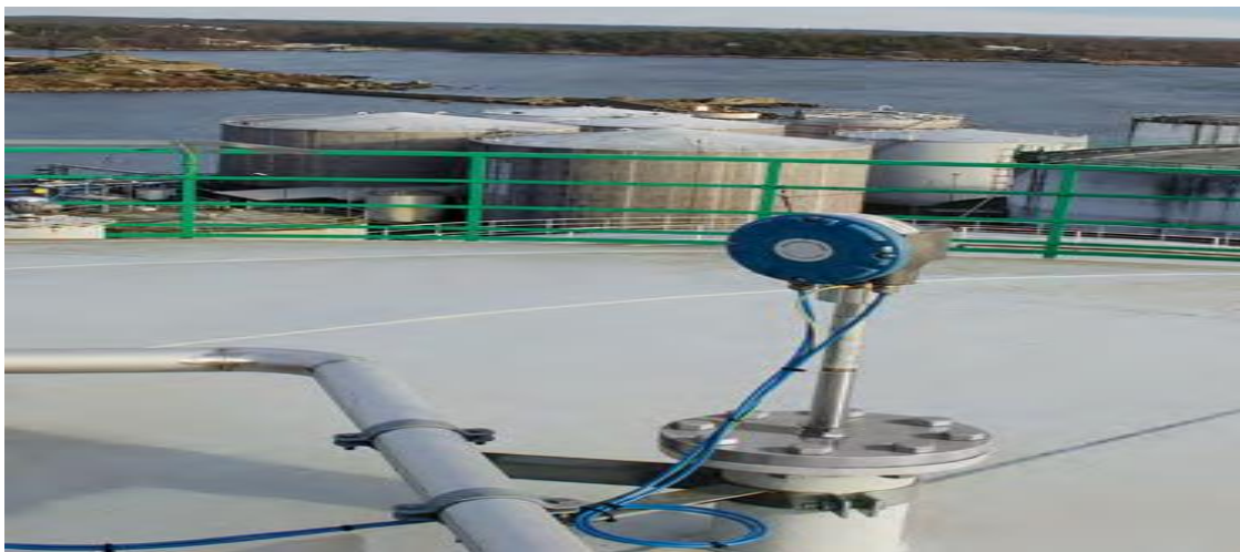
Plate 2.1: Top mounted temperature transmitter for up to 16 spot temperature elements (Devold, 2013).
