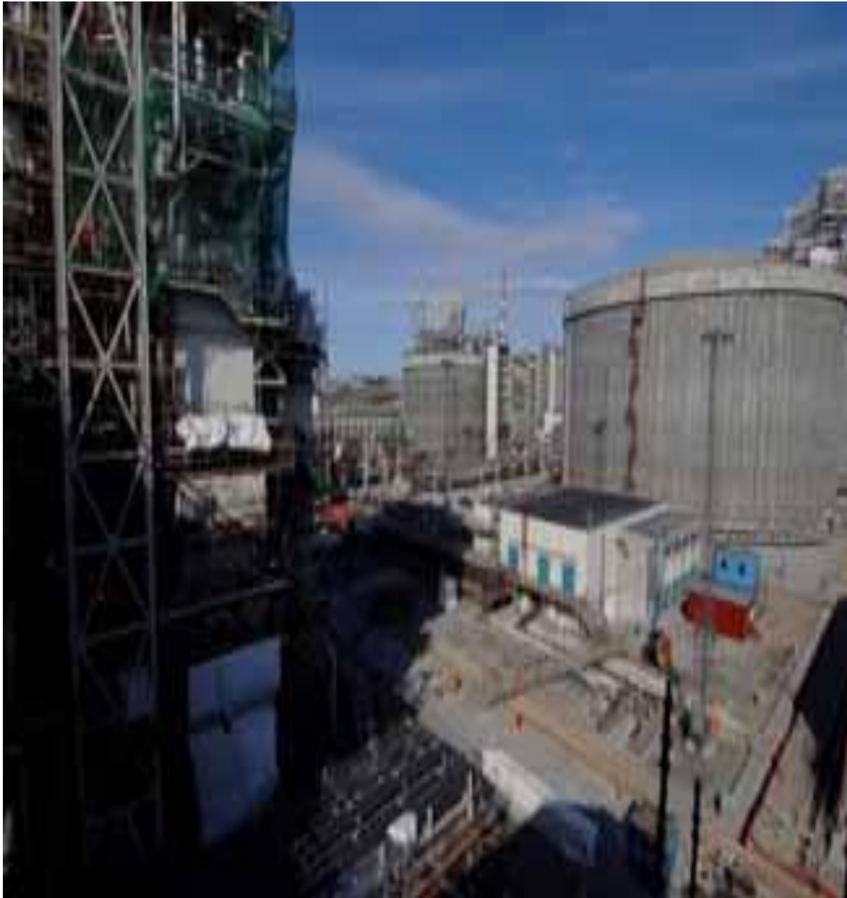
Plate 1.1: Typical Process Facility and Storage Tanks (Devold, 2013).
