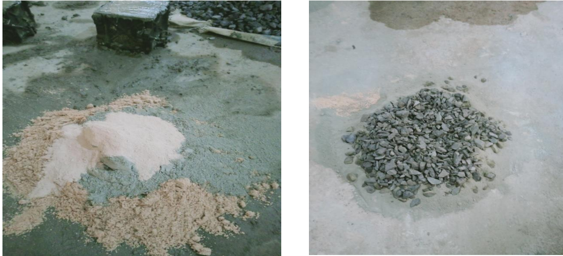
Plate 3.9: Mixing of binary concrete
