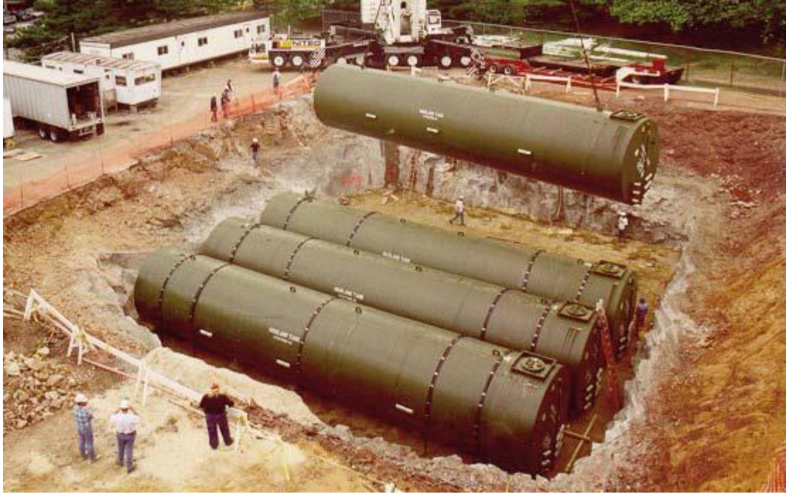
Figure 2.3: A typical UST installation
