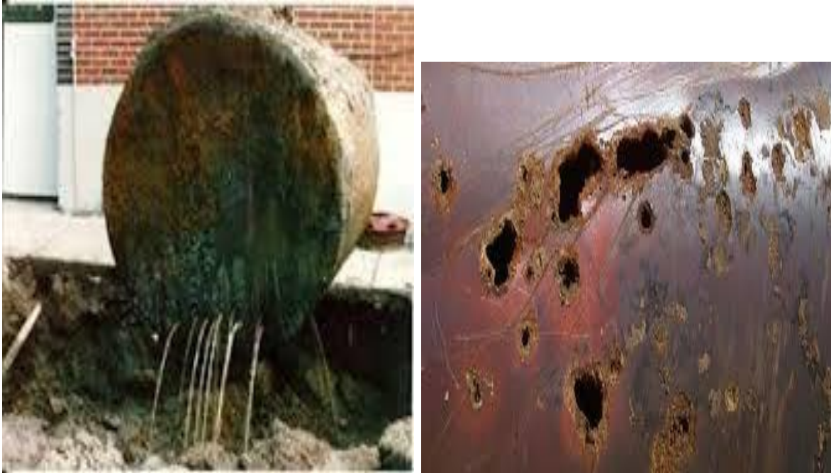
Figure 2.4; Fuel leakage from a corroded UST; Source: DEFRA 2000
