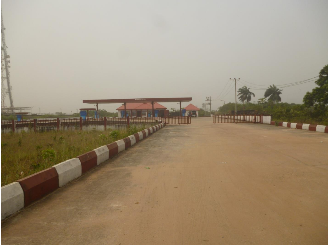
Integrated petrol station: properly situated
