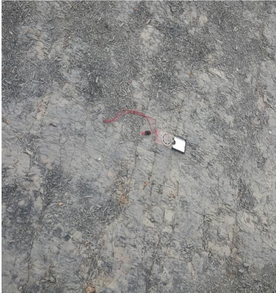
Figure 4.33: Faulted Shale (UTM zone 32: Lat 982403, Long 658025)
