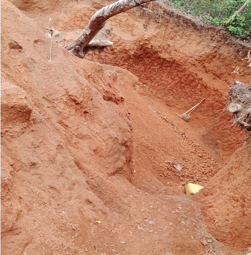
A pictorial view of a rocky ground where quarry works is done as captured by the Researcher.
