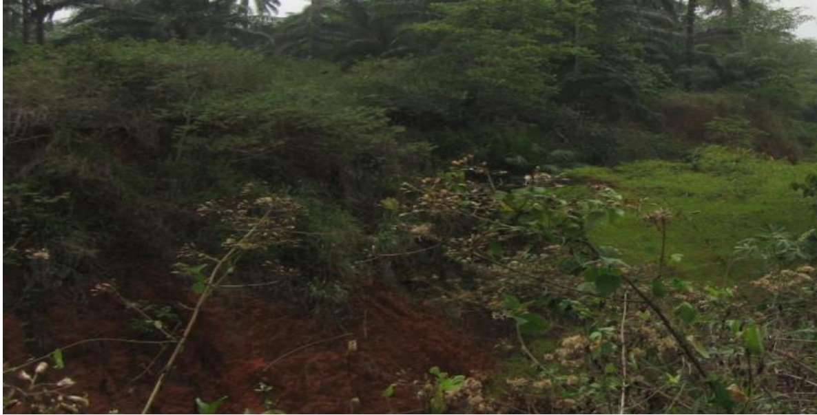
Appendix 1a: showing secondary erosion channel
