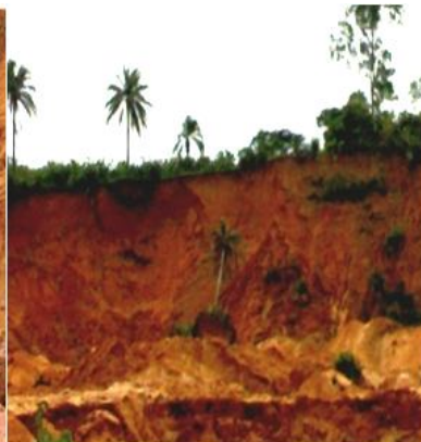
Plate 3a: Abandoned borrow pit showing old slide surface and recent slumping b: Active borrow pit with rapid sliding and palm trees hanging next to pit crest often sliding and causing damages to the excavator c: Heavy duty excavator at work
