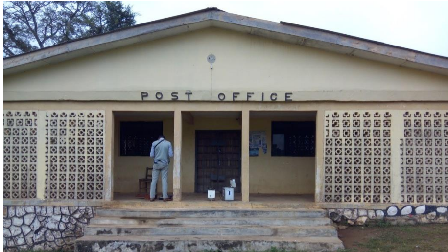
Igbara-oke post office
