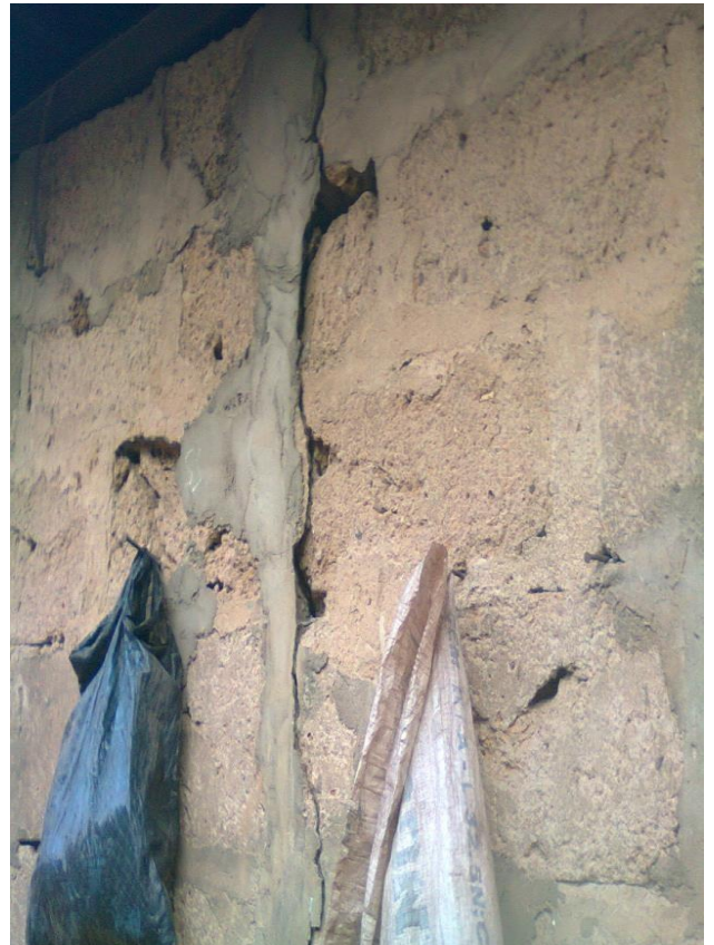
Plate 4a: Cracked buildings within Lokpaukwu area (study location)
