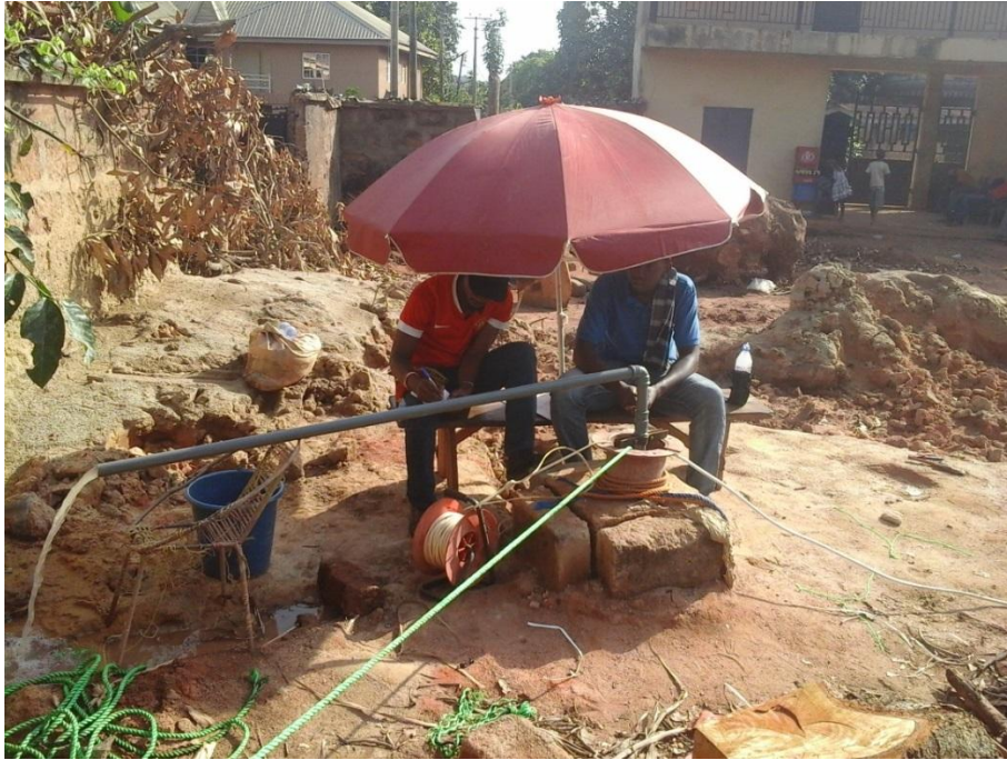
Figure 3.1: Pumping test ongoing
