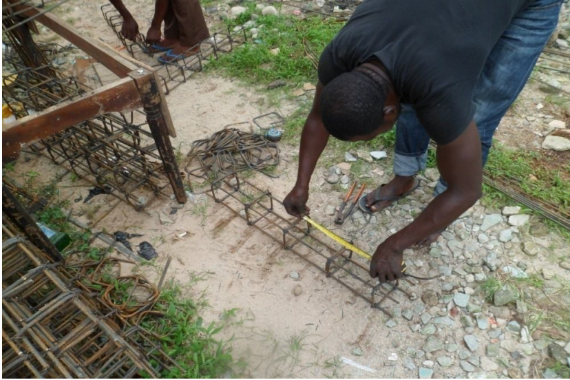
Plate A.2 Measuring and Fabrication of Conventional Reinforcement
