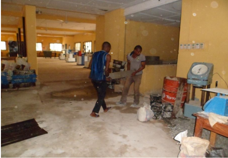
Plate A.11 Carrying of beam to an open curing tank
