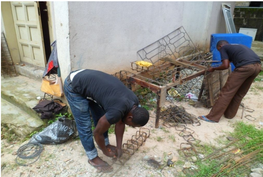
Plate A.3 Fabrication of Conventional Reinforcement.
