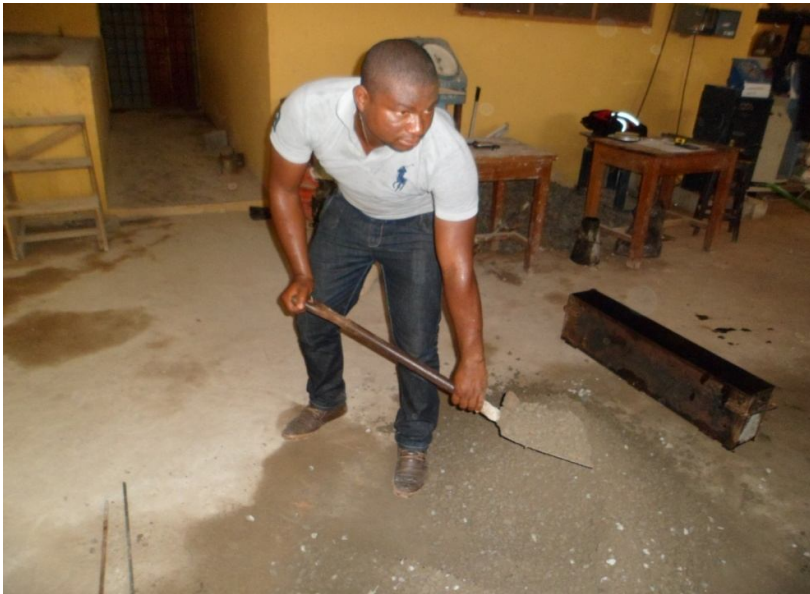
Plate A.7 Mixing of Concrete
