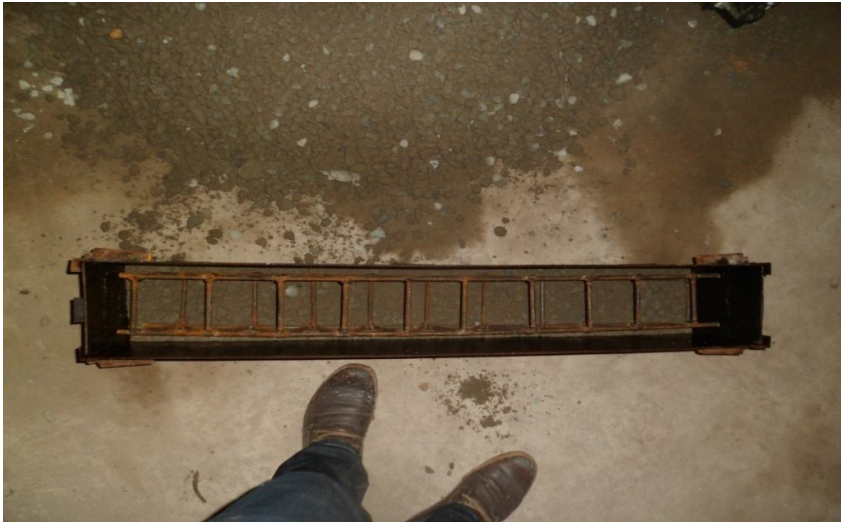
Plate A.8 Truss Reinforcement Beam well positioned inside Beam Mold
