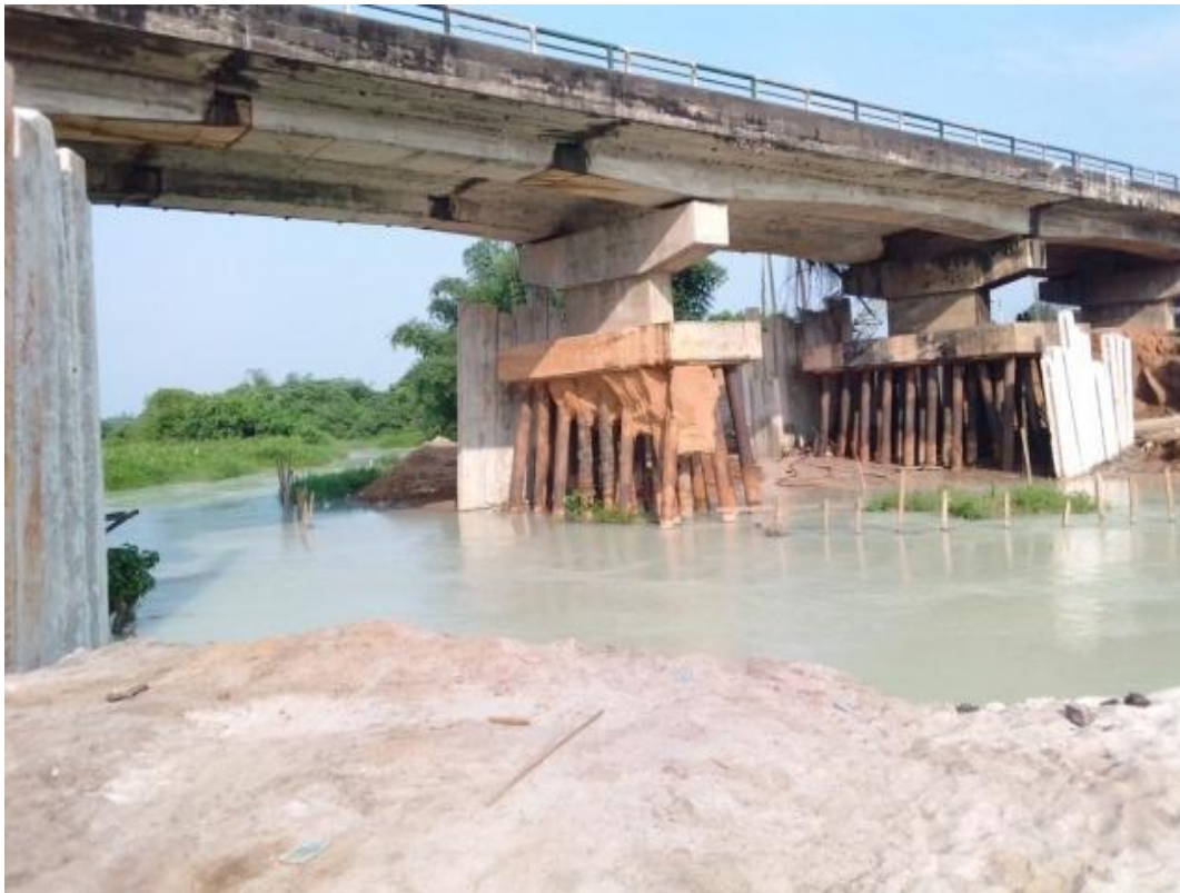
Photo showing the effect of sand dredging on Otamiri River on FUTO Bridge
