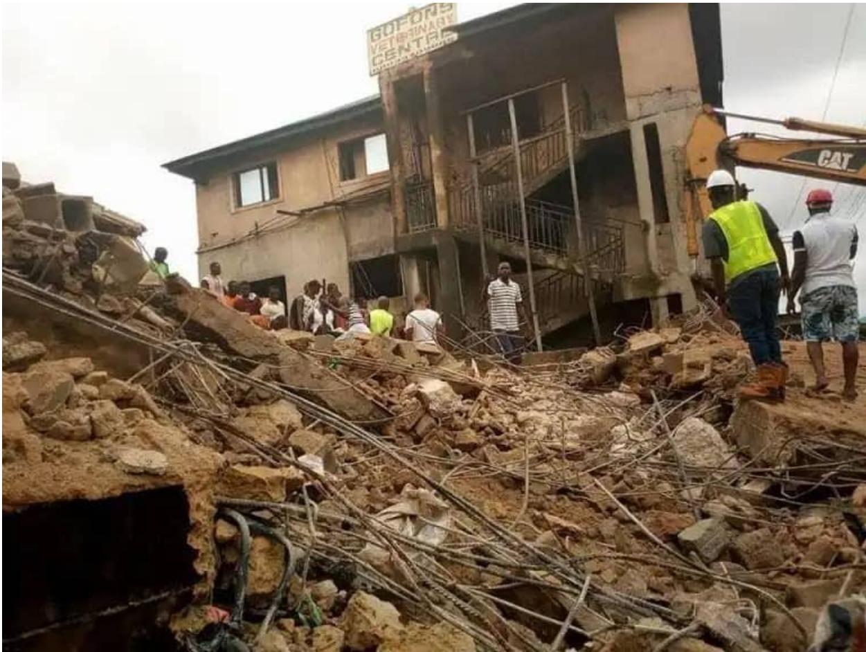
Plate 8: Collapse of a Two Storey Building around Fire Service Area/Mbaise Road, Owerri, 2017
