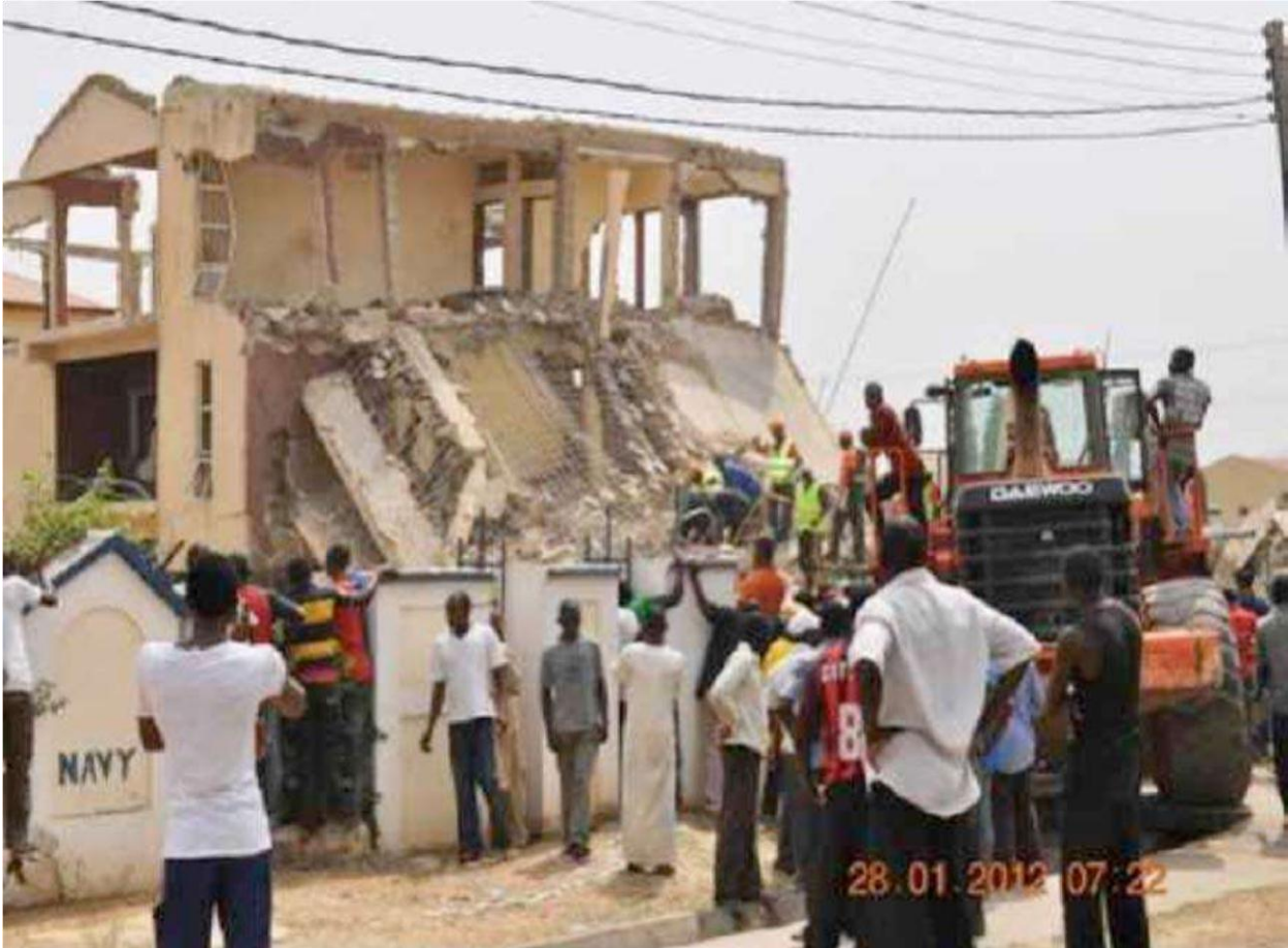
Plate 1: Collapse of Two storey Naval building in Abuja ( Source: Ebihikhalu and Dawan, 2014)
