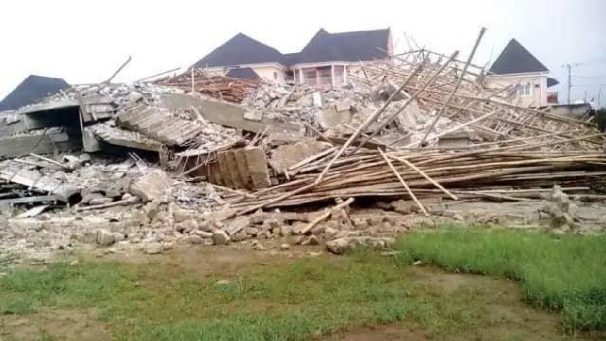
Plate 7: 3 – Storey Building that collapsed in Umuguma, Owerri West LGA, 2018. Source: www.google.com.ng
