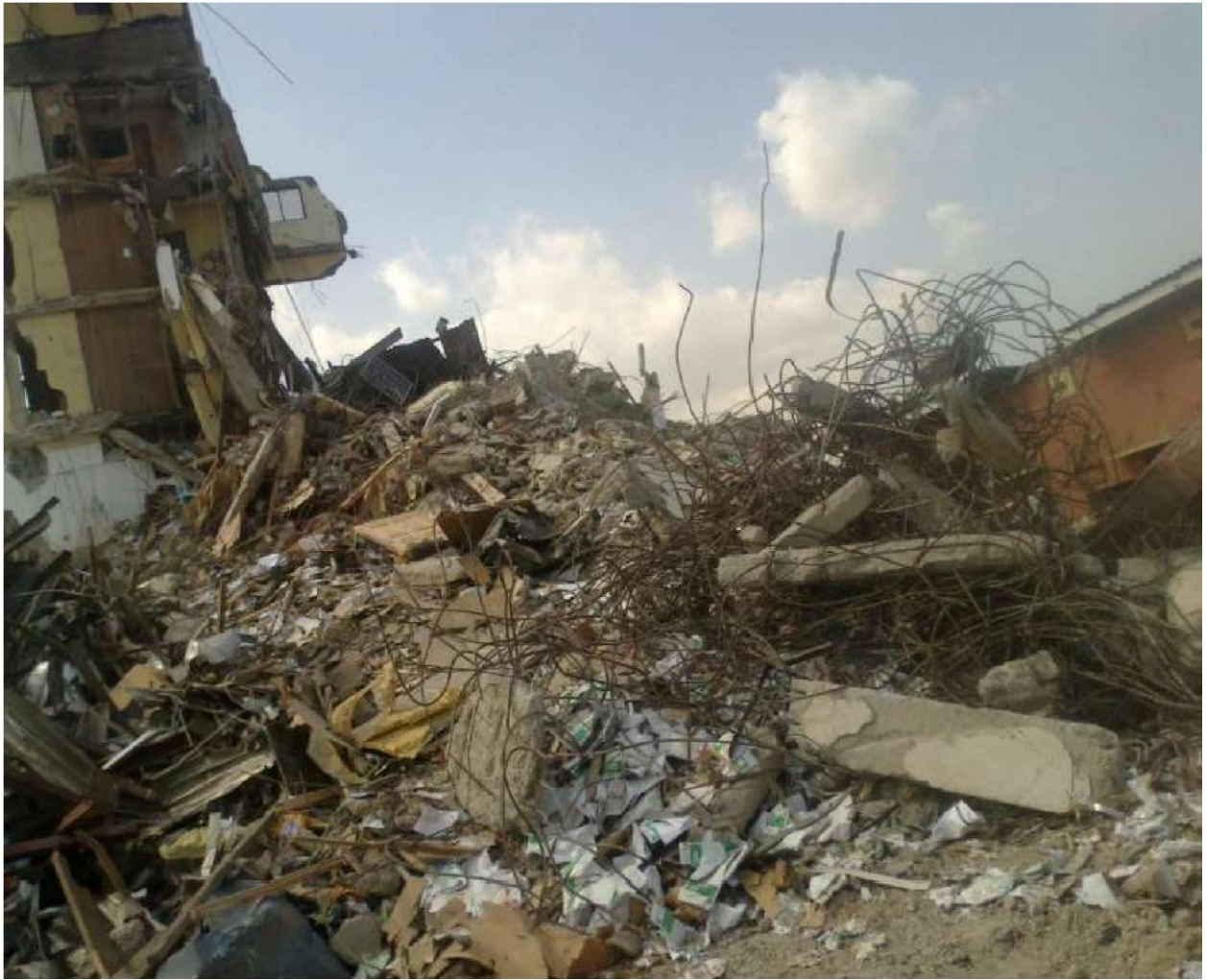
Plate2B: Six Storey building at 11 Aderibigbe Street, Maryland Lagos (Source: NBRRI)
