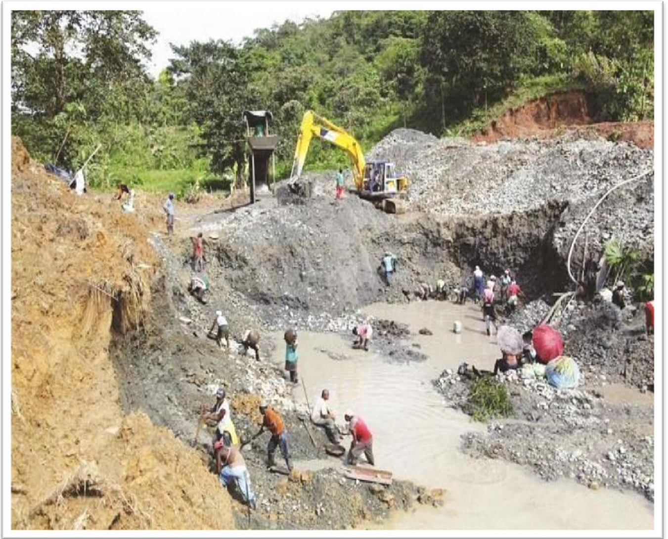
Plate 3.1: Sand mining along Onuiyieke River at Ogwogoroanya (near Site Location 3)
