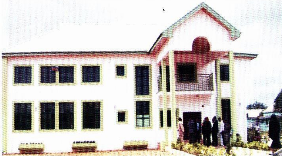
The newly constructed FUTO Consult Office.
