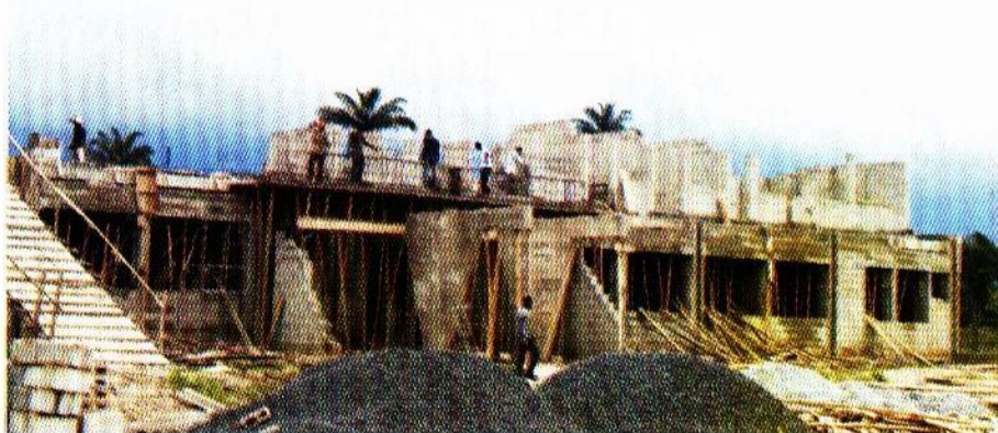
The School of Environmental Sciences and Technology building under construction.
