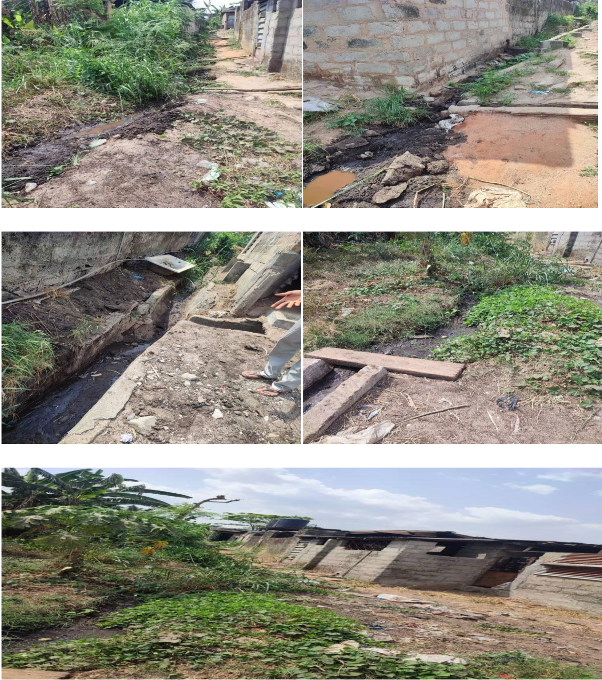
Plate 3.1: Pictures showing the channels through which untreated pig wastewater are discharged from the farm to a nearby river
