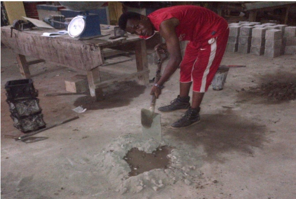
Plate B.6 Mixing of Concrete Materials
