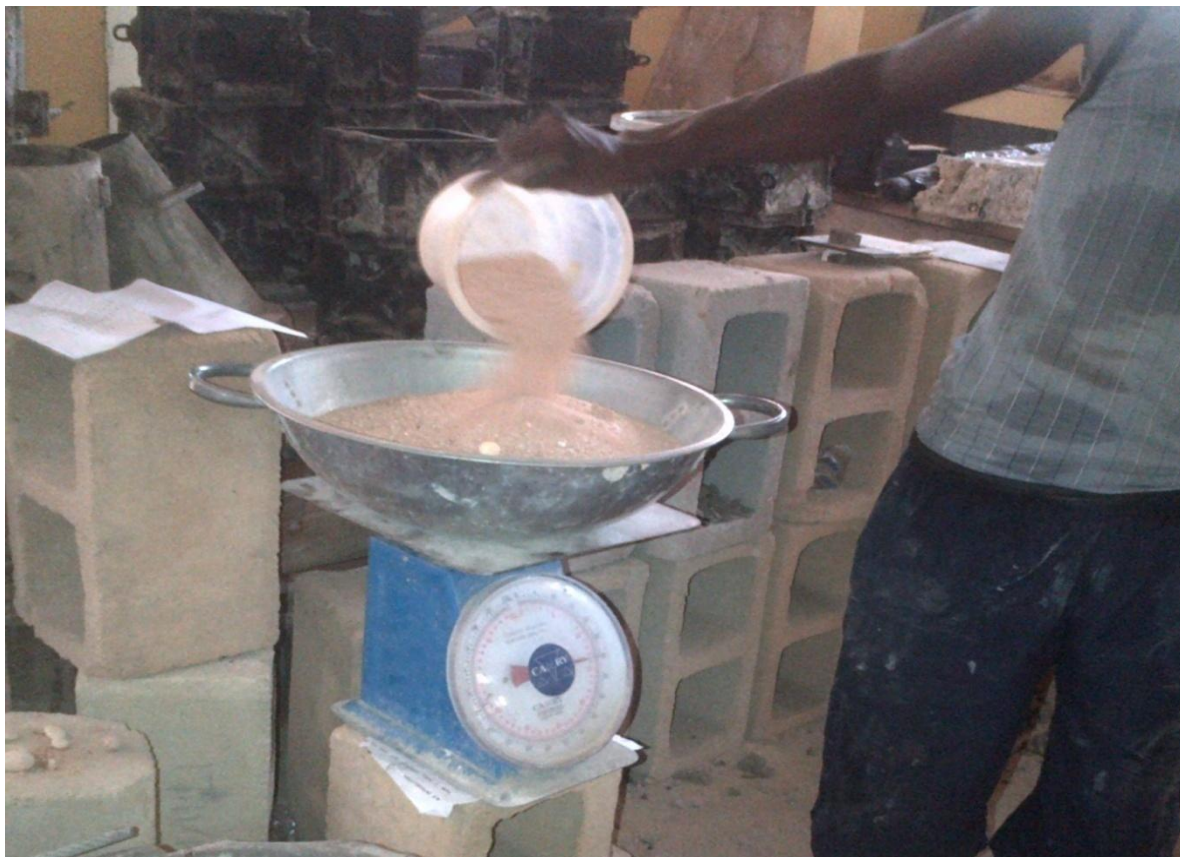
Plate B.2 Batching of Sand
