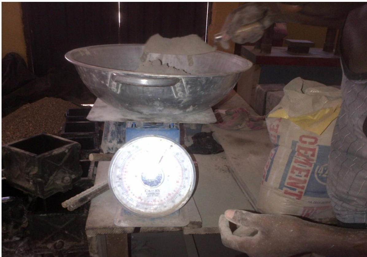
Plate B.4 Batching of Cement
