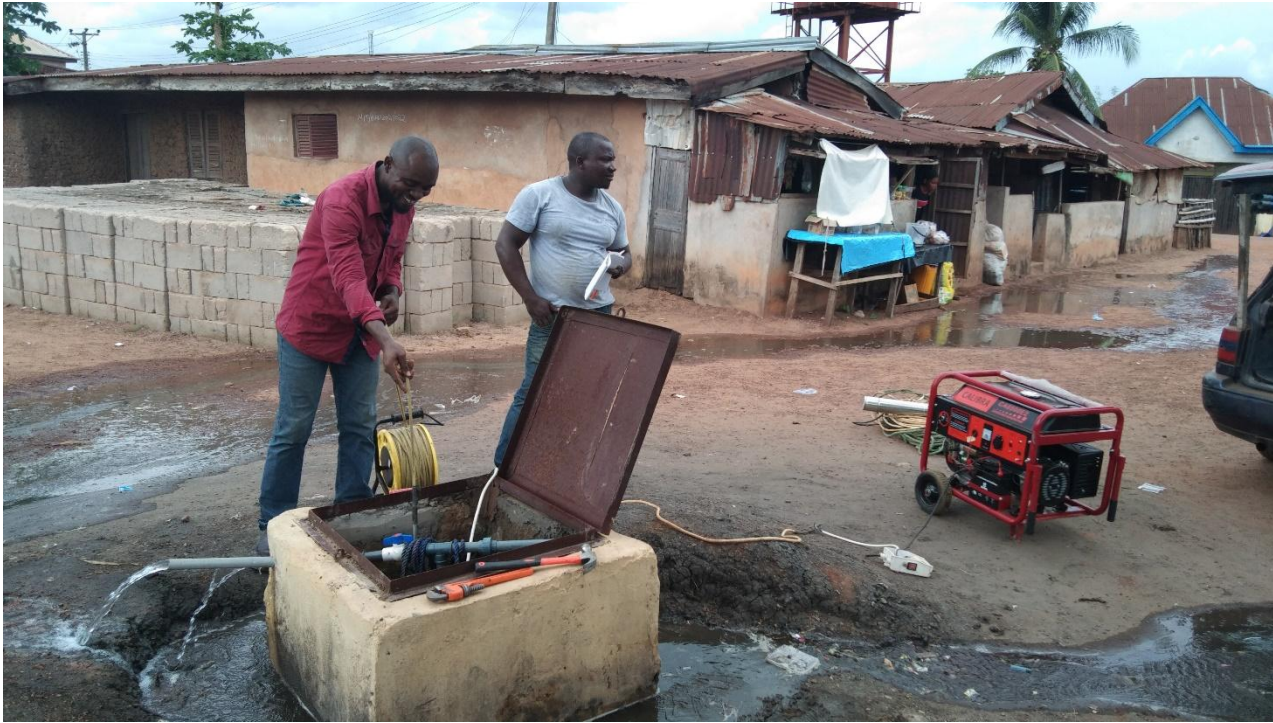
Figure 3.1b: Field Pictures of Pumping test in the study area by Constant Rate Tests
