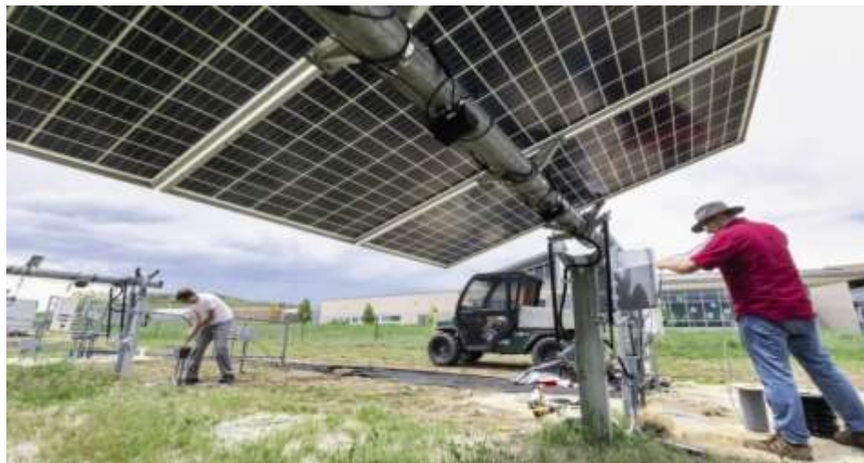
Plate 2.8: Field installed BFPV module. Source: Sng et al., 2021
