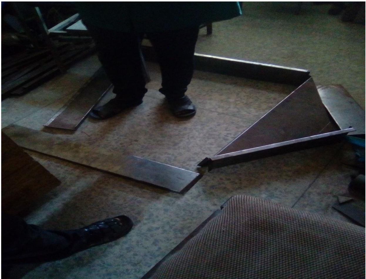
Plate 10: Assembling of the soil bin
